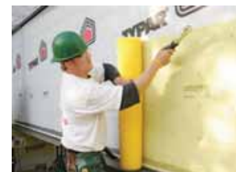
Courtesy of APA – The Engineered Wood Association
