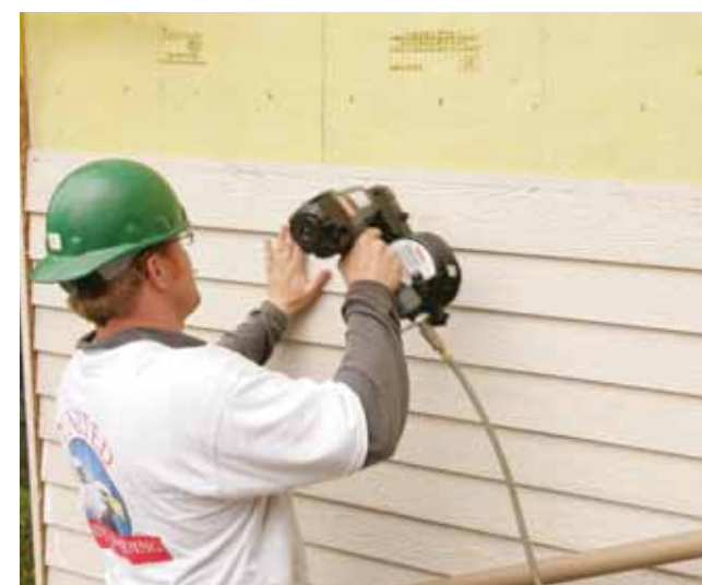
Courtesy of APA – The Engineered Wood Association
